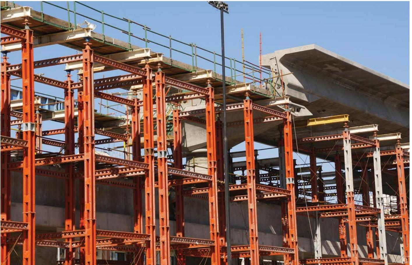
So colossal has been the scale of the scheme which VFR is undertaking that the consortium had up to a dozen sections of the route under construction at any one time; with RMD Kwikform being called upon to supply Megashor towers to site for erection within a very short time frame.
