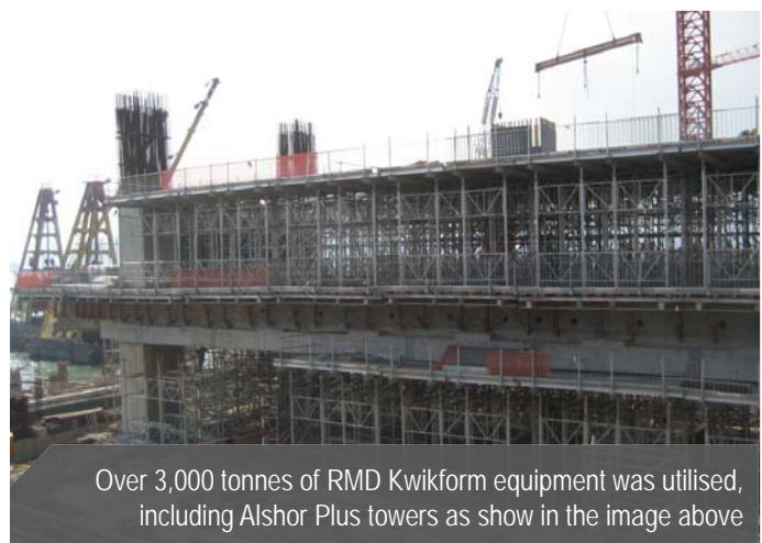
Construction of Kai Tak Cruise Terminal
