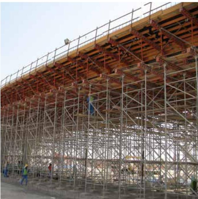
In order to cut programme time down to a minimum, in addition to using the Rapidshor system, RMD Kwikform engineers also designed the cantilever footway sections of the bridges as standard units that could be pre-assembled on the ground prior to erection on site. Anvar: "By standardising the cantilever sections for all the varying super-elevations we were able to reduce the need for more complex assembly and ensure quality of construction and erection was maintained.
